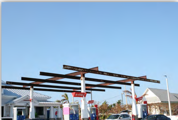
A gas station with its roof torn off near Key West and Hawks Cay Resort.
