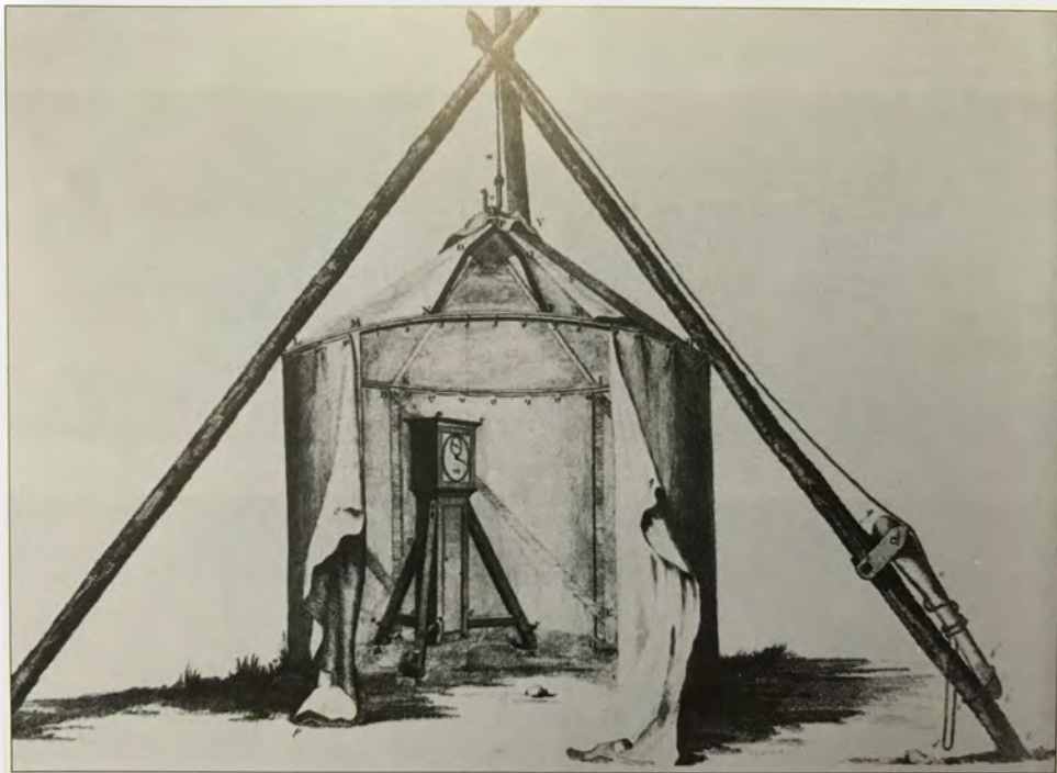
Mason and Dixon's observatory at the Cape of Good Hope was constructed of canvas, wood, and bricks and did more than just shelter their instruments. It also provided them with a stable base from which to make their observations and measurements. The observatory pictured here is similar to the one they built.
