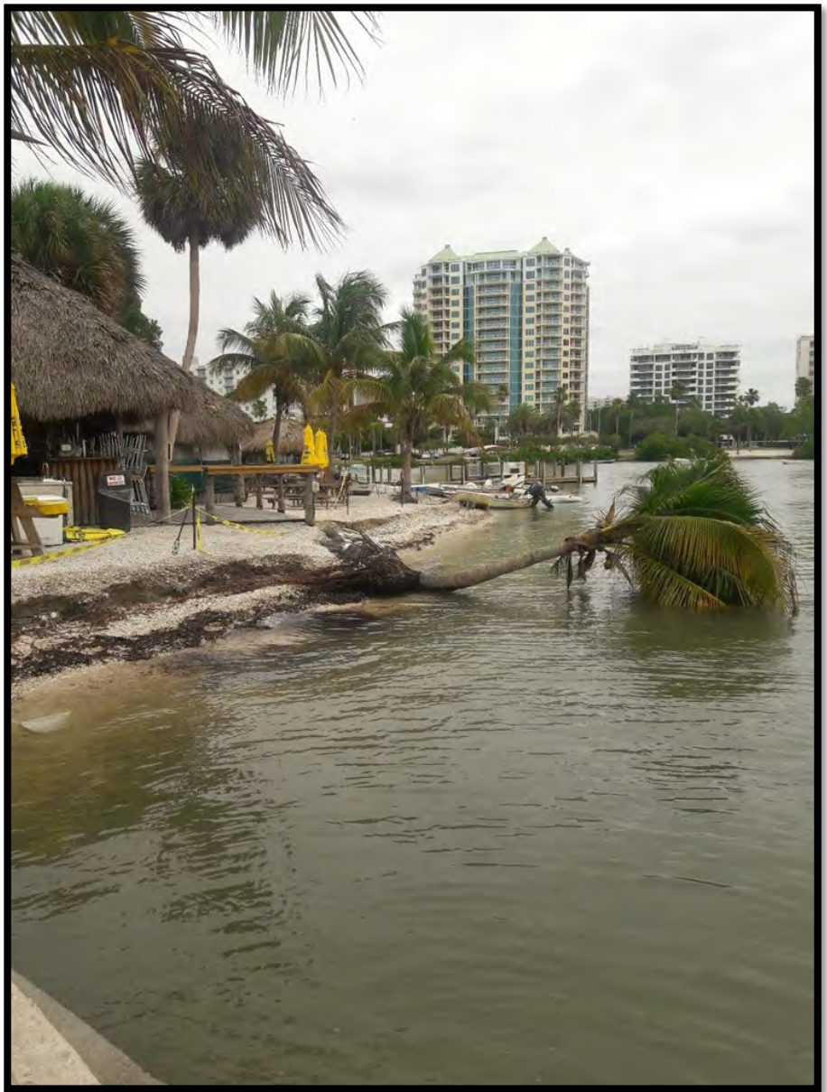
Storm damage sustained in May 2017 only weeks prior to the start of construction, causing the need for a FDEP permit modification to place fill prior to installation of the sheet piles.
