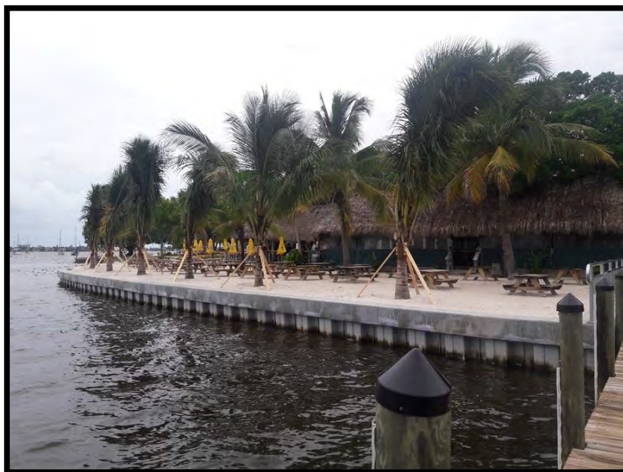
Traditional seawall days after the passing of Hurricane Irma in August of 2018.
